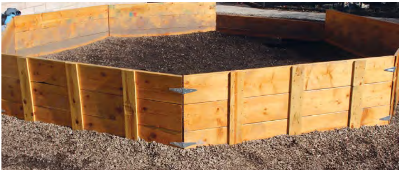
Ga-ga pit constructed in the Falk Wonder Lab.
